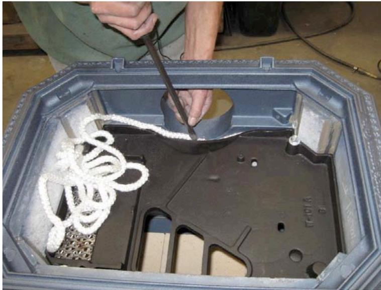
5. Apply a bead of stove cement over the top of the new gasket. Use your finger or putty knife to smooth the cement. Wash hands and tools with warm soapy water.
