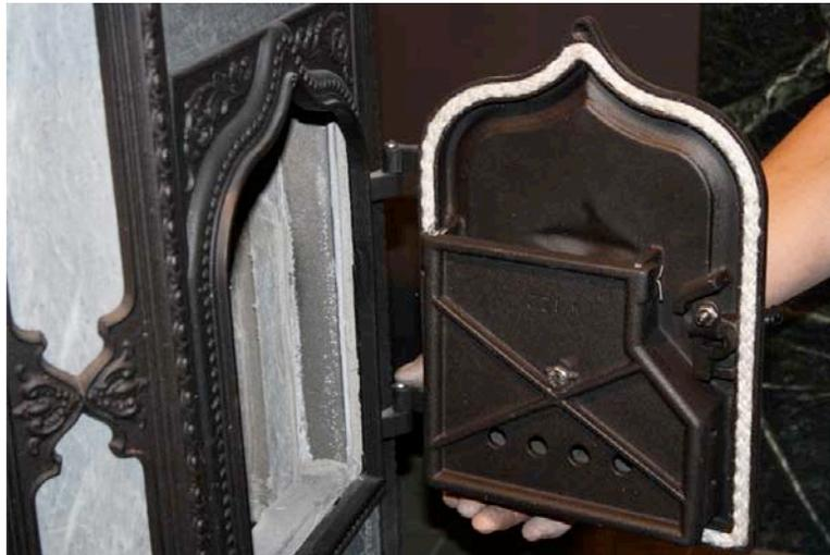
3. Lay the door face down on a suitable work surface. Use a putty knife to remove the old gasket. A wire brush may be used to clean out any cement residue from the gasket channel. Vacuum any leftover debris from the door and gasket channel.
