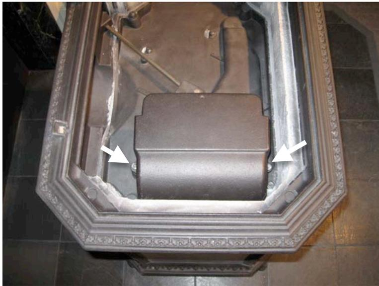
3. Use a putty knife to remove the old gasket from around the perimeter of the hood. Remove any residual gasket and furnace cement with a wire brush and vacuum.
